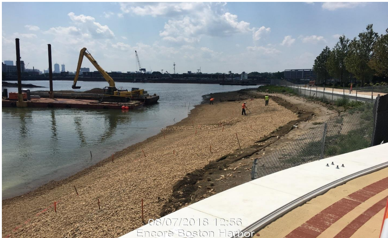
Photograph #2: Nearing completion of dredge cap repair work, eastern shoreline of Site.
